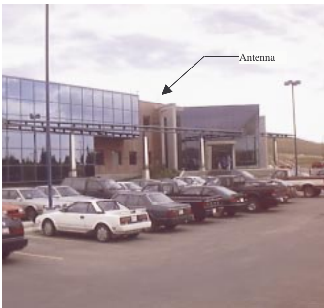
Figure 11: Antenna array on the roof at NovAtel Inc.
